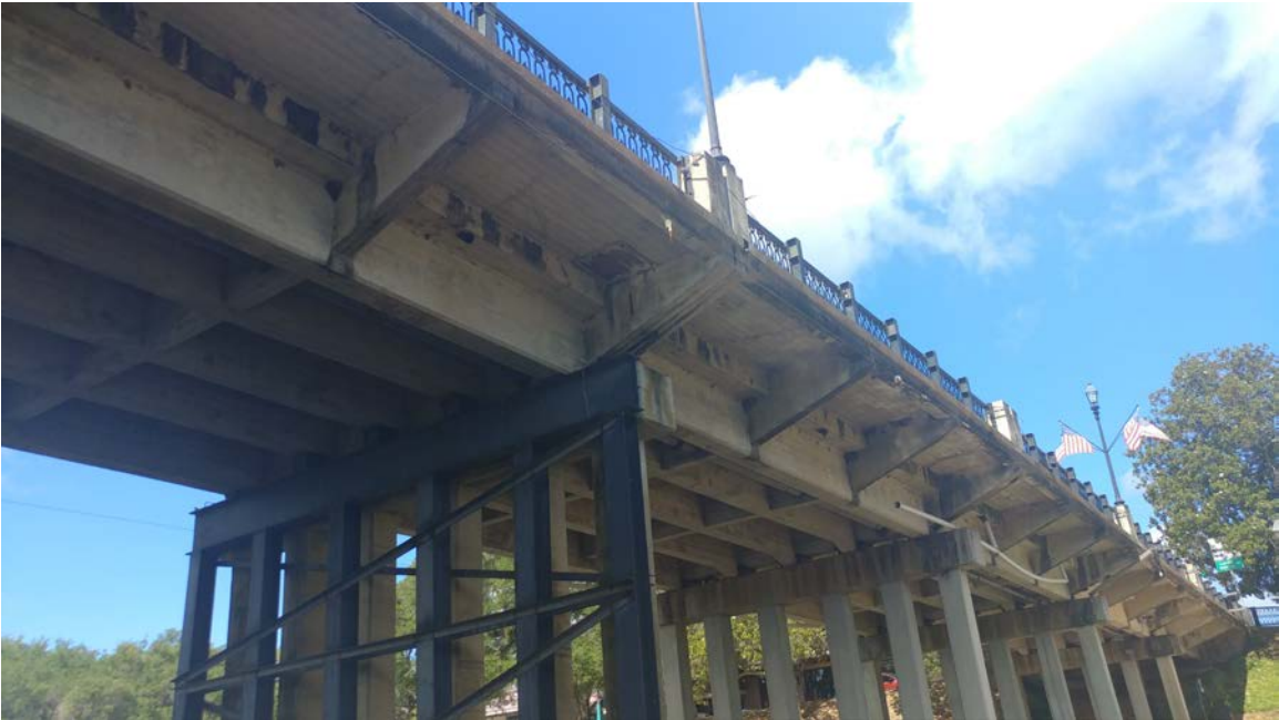
Photo 10: View of existing bridge at Church Street
