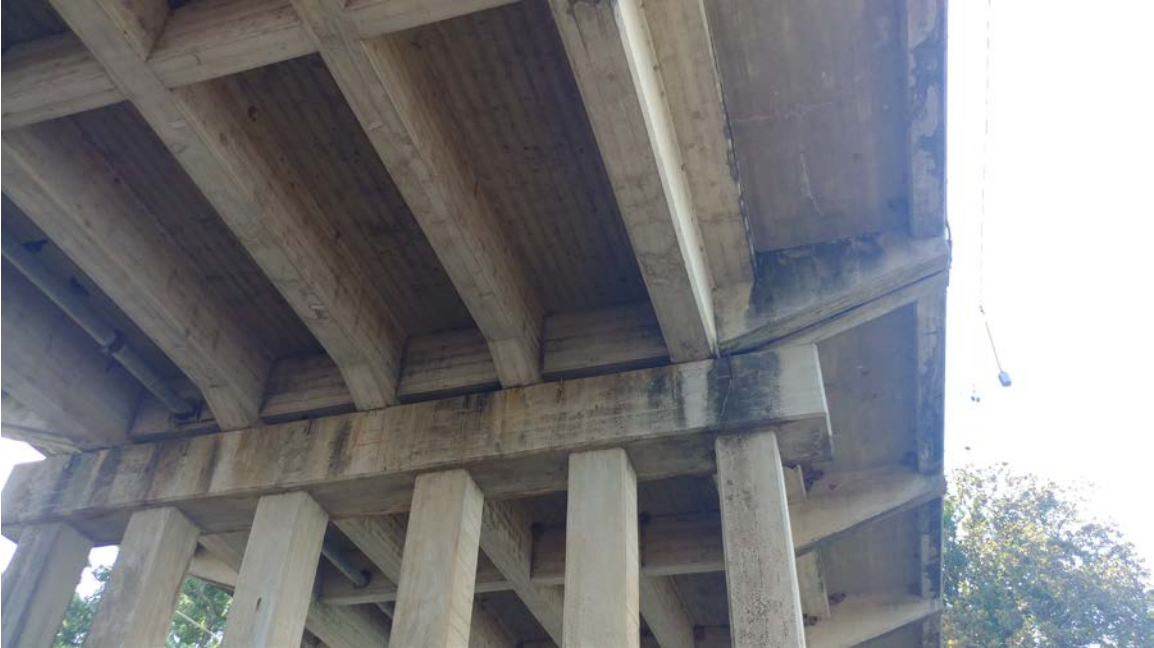
Photo 11: View of existing bridge at Church Street
