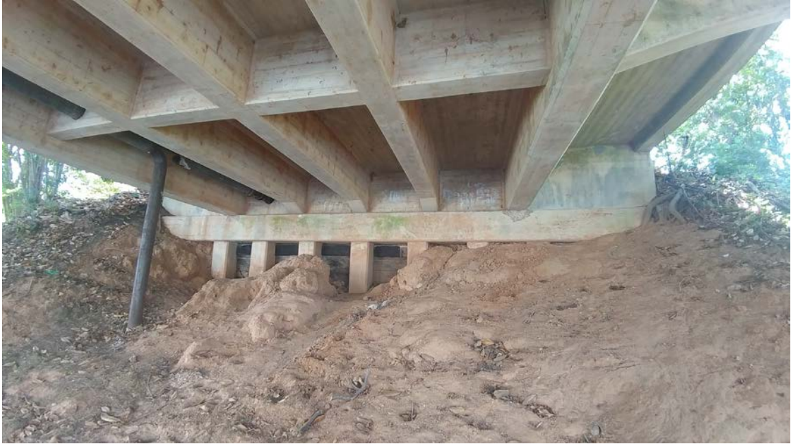
Photo 9: View of existing bridge at Church Street
