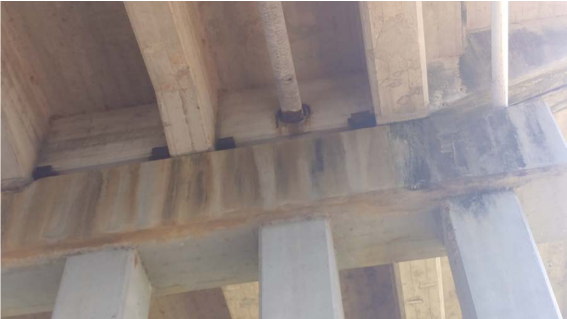
Photo 12: View of existing bridge at Church Street
